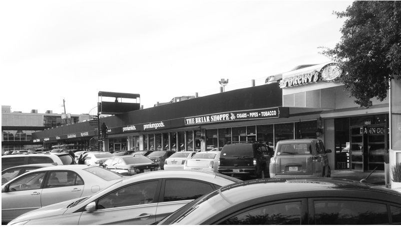
Figure 17: Rice Village, Houston. Note the parking on the roof.
